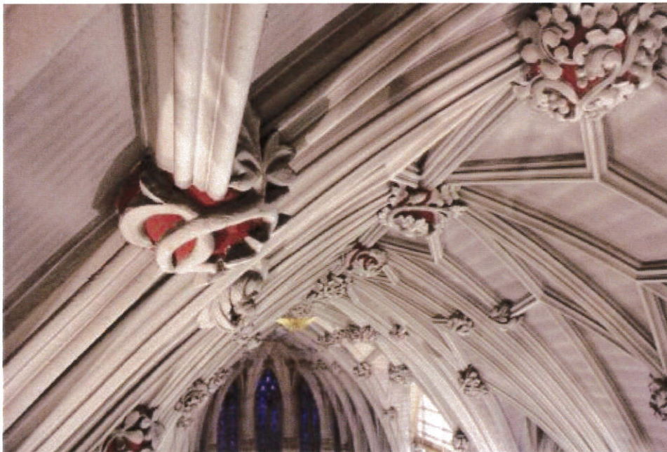
Each of the red decorative bosses that adorn the ceiling have a unique design. The plastered ceiling vaults will soon be scrubbed clean and repainted.
