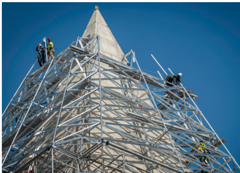
From 500 to 555 ft. a 70-ft.tall, fabricated aluminum structure crowns the structure’s Pyramidion.
