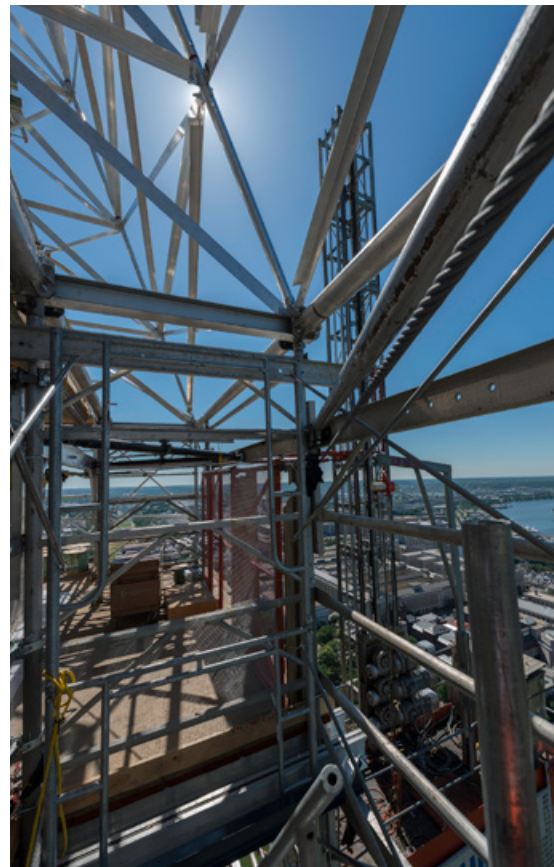
At the base of the Pyramidion the angle of the scaffold tilts, going from a 1° to 17° taper all the way to the top of the structure.
