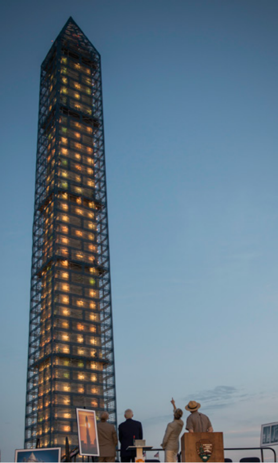
The scaffold, wrapped in decorative scrim and lights, was lit July 9, 2013.
